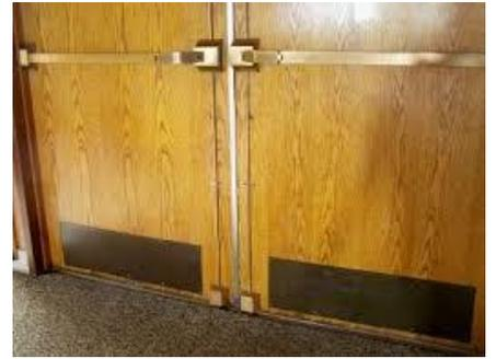
**PULL SIDE Standard SAFETY Guard** installs the same with panic-bar doors, no WIDE for Pull-Side necessary
